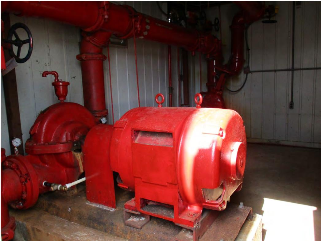
Photo 6: View of AFFF pump and pump controller at Hangar 985.
