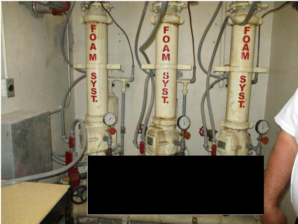
Photo 4: View of AFFF fire suppression piping at Hangar 985.
